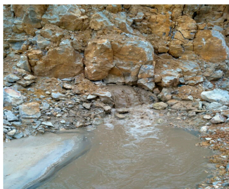
FIGURE 13 Photo of leakage at the water inflow point during K373# grouting.
