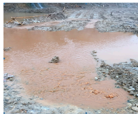
FIGURE 14 Photo of leakage at the water inflow point during K485# grouting.
