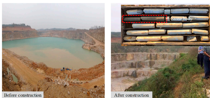
FIGURE 15 Comparison of the effect of core sample and limestone mining area water inflow treatment after grouting before and after grouting construction.
