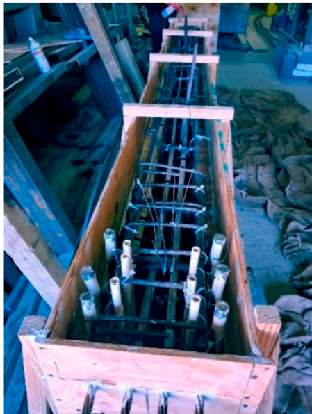
FIGURE 18 Reinforcement layout.
