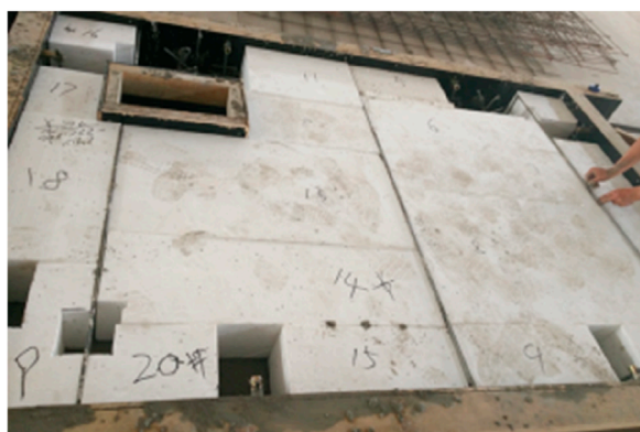
FIGURE 4 Installment of the insulation board.
