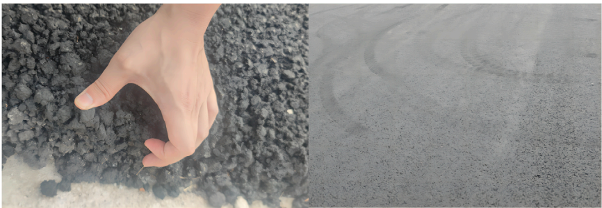
FIGURE 1 Loose and rutted new asphalt pavement.
