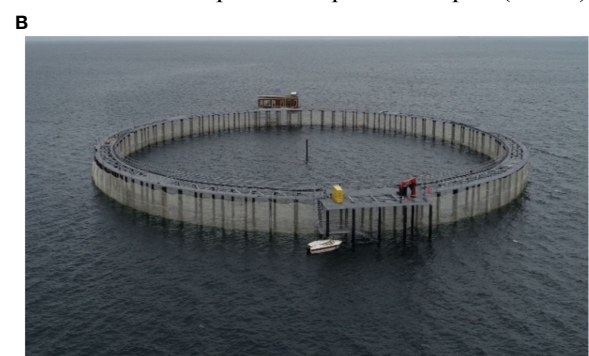
coast-connected pile-net aquaculture pen (CPAP)
