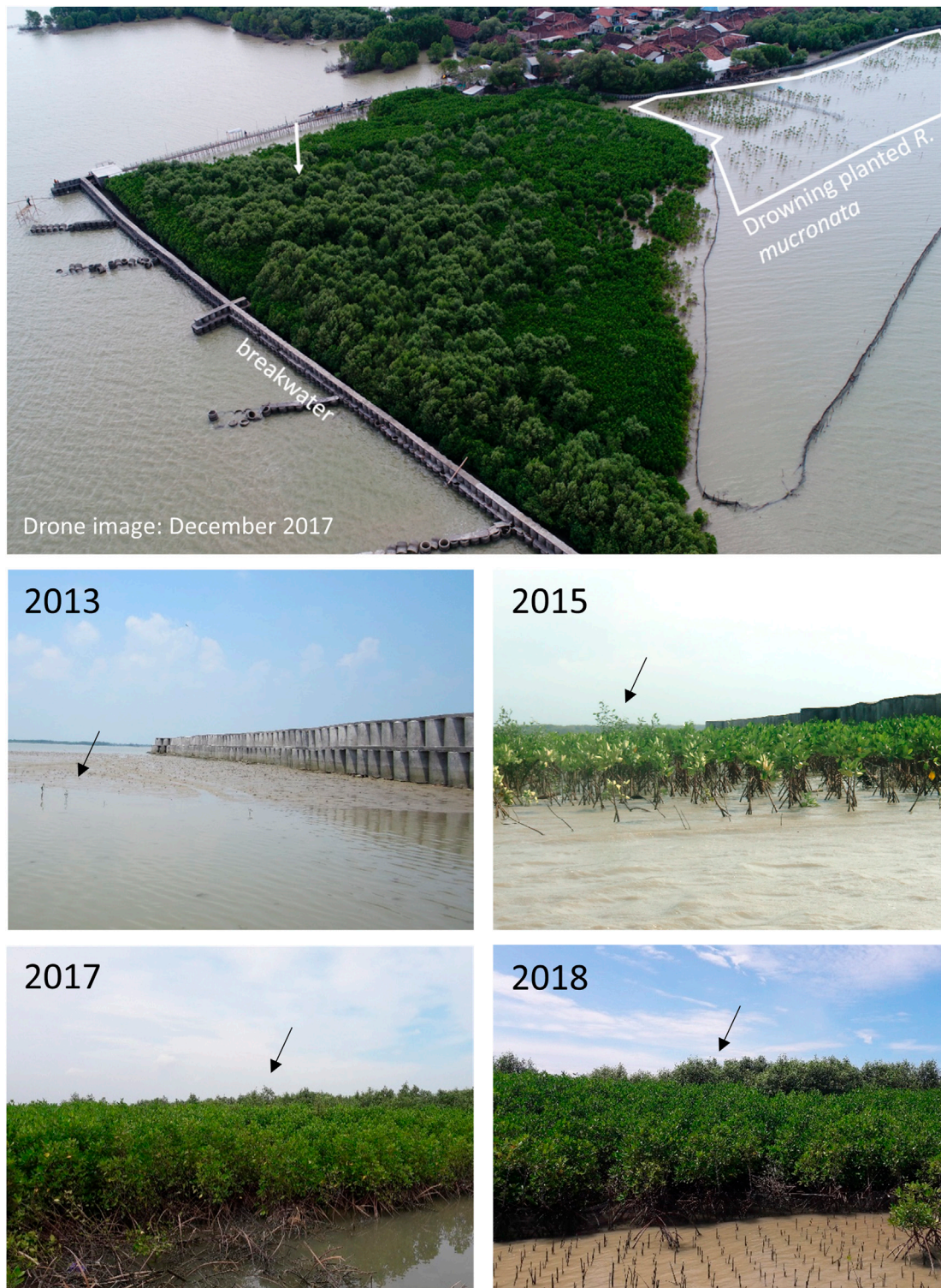
FIGURE 9 | Top: Bird's-eye view of the breakwater seaward of Wonorejo, Demak in 2017 (drone image courtesy of CoREM-UNDIP). The white arrow indicates the direction of the picture time series. The time series show the development of a mudflat after construction of the breakwater in 2012, followed by natural colonization in 2013 and subsequent planting of R. mucronata in 2014. Note the relative height difference in all pictures of the naturally colonized A. alba trees (black arrows) versus the surrounding planted R. mucronata trees (2015–2018).
