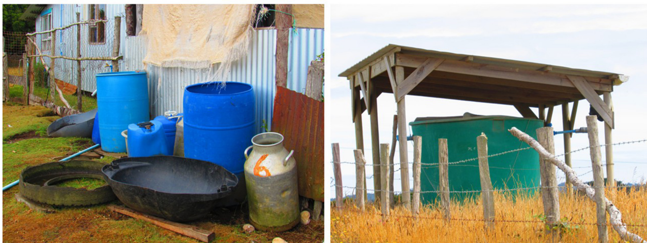
FIGURE 4 Examples of rainwater harvesting systems present in Ancud, Archipelago of Chiloé. On the left, an improvised system made with recycled materials; on the right, a mechanized system. Source: Photograph by the Authors.
