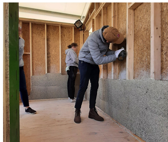
FIGURE 3 Single-sided hempcrete forming against wood sheathing, successfully used by the author and his students in a 2023 project (Source: Author).
