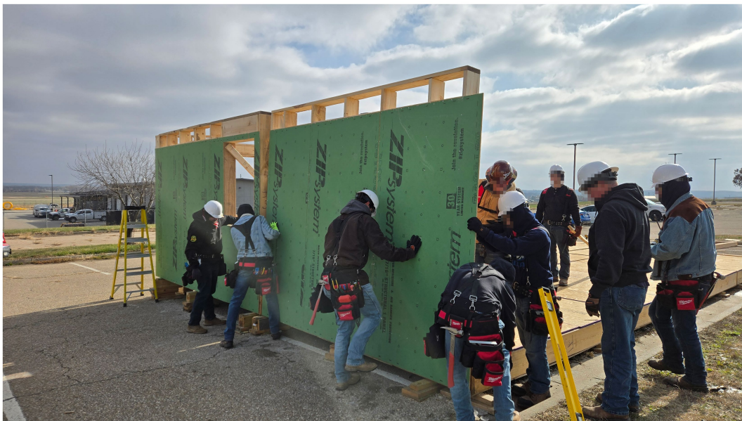
FIGURE 10 Students from Manhattan Area Technical College (MATC) erect wall panels at the K-State College of Architecture, Planning, and Design's off campus shop (Source: Author).
