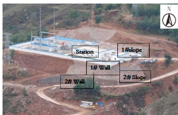
FIGURE 1 Image of the transformer station.
