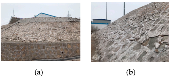
FIGURE 9 Drainage hole. (a) Drainage hole on the south slope. (b) Drainage hole on the north slope.
