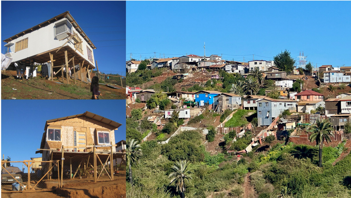
FIGURE 3 Construction typology of housing in the settlement Felipe Camiroaga, Viña del Mar. Source: Authors.
