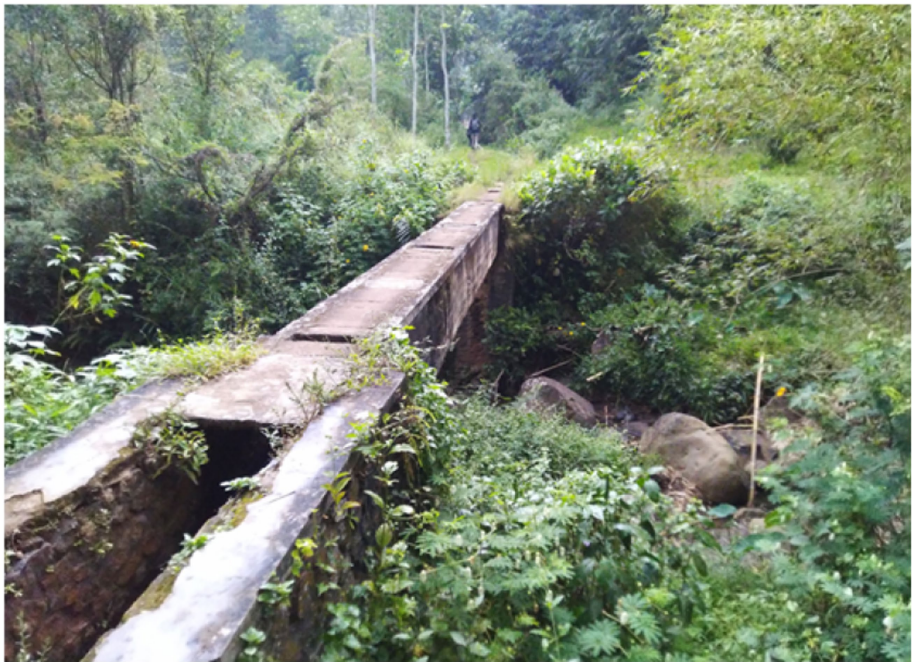
FIGURE 5 Dry irrigation channels. Irrigation flows from Sawah Valley Watersprings toward the agricultural lands of Wagir District.
