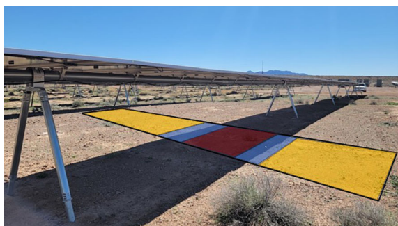
FIGURE 3 Panel microsite locations at Gemini. Yellow = interspaces between panels. Blue = panel dripline. Red = under panel.
