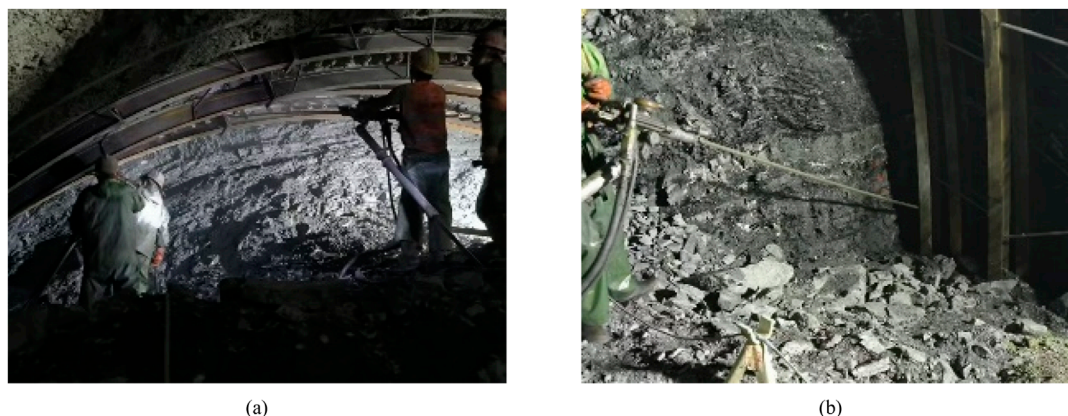
FIGURE 14 Test section site construction drawing. (a) Workers are applying an overrun small conduit. (b) Installation of foot-locking bolts.
