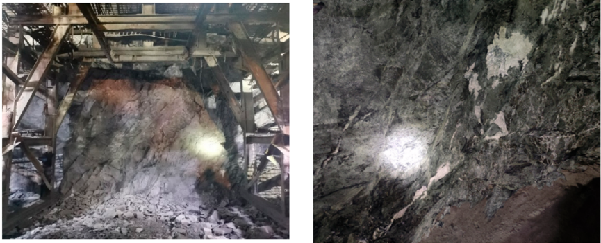
FIGURE 11 Site photograph of the excavation face in the Class III surrounding rock tunnel section.
