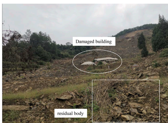
FIGURE 4 The whole picture of landslide impact scraping area.
