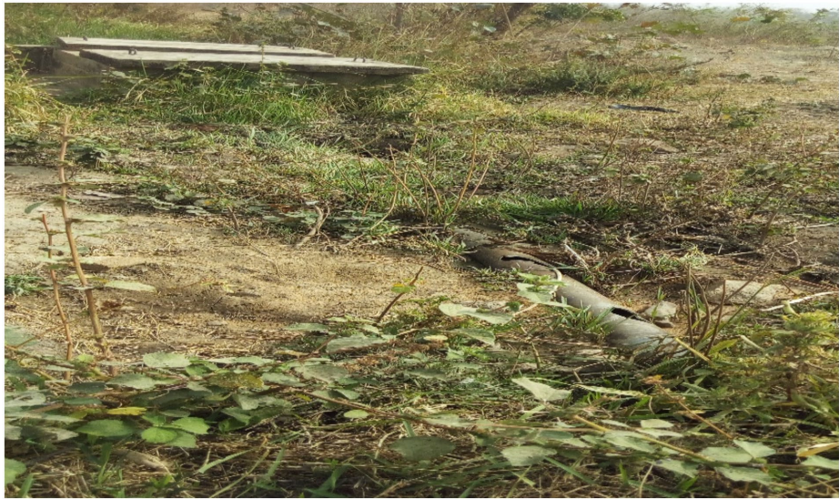
FIGURE 2 A broken irrigation water supply pipe at the Nyimati community irrigation site. Source: Field Survey, February 2024.
