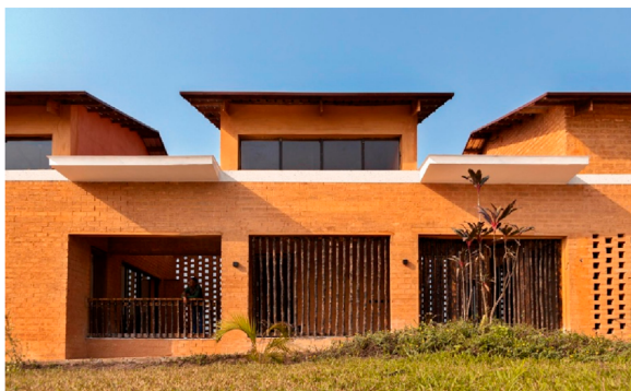
FIGURE 1 Ecology Green Farm "earth brick barn house" designed by MOE + Art Architecture for Yinka Shonibare Foundation, southwestern Nigeria (photo: Andrew Esiebo/Wallpaper).
